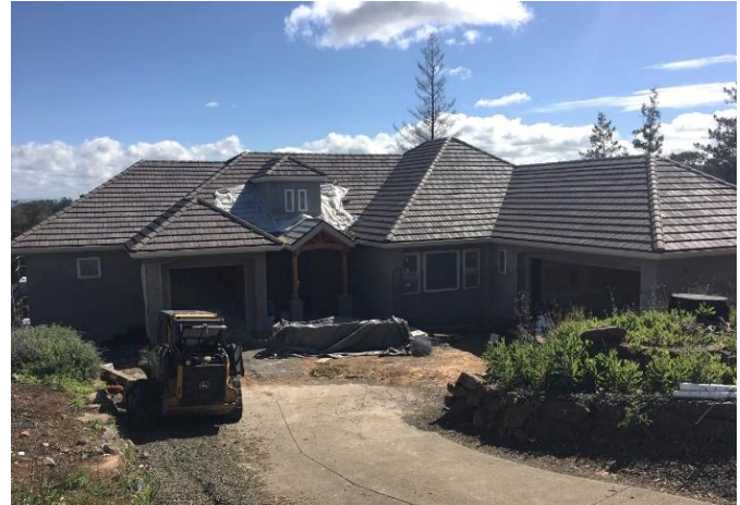
Figure 1. Home undergoing construction
