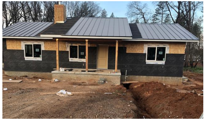
Figure 2. Street view of the rebuild under construction
