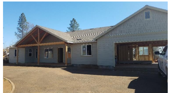
Figure 2. New home under construction
